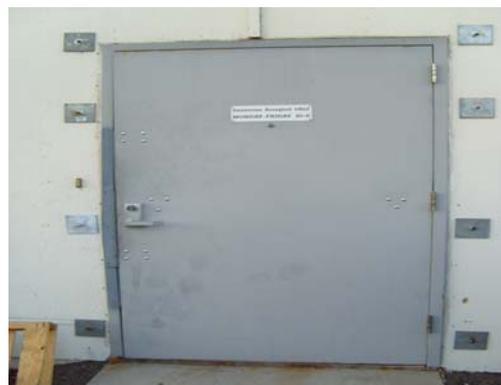
the spike and even the fork end of the halligan can be placed on top of the hinges and struck to remove them from the hinges. Know your tools ~even though the rotary saw/ K-12 is the fastest a set of Irons with the knowledge to use them are still the keys to any door. 🔥
